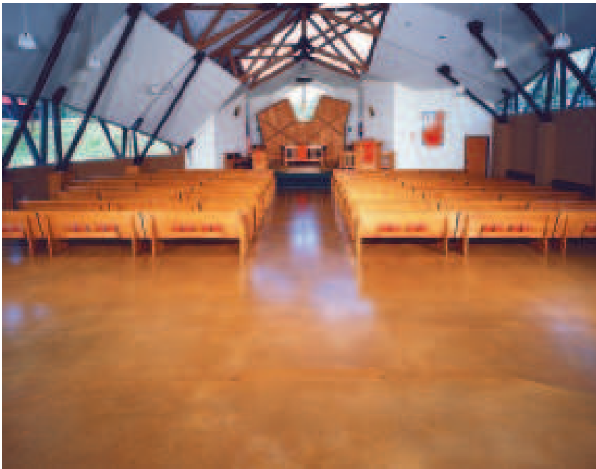
Water-based acrylic sealers are a good choice when sealing indoors, especially in areas that will be in use during the job.
