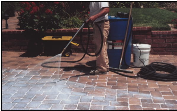
Learn how to clean and seal paving projects
